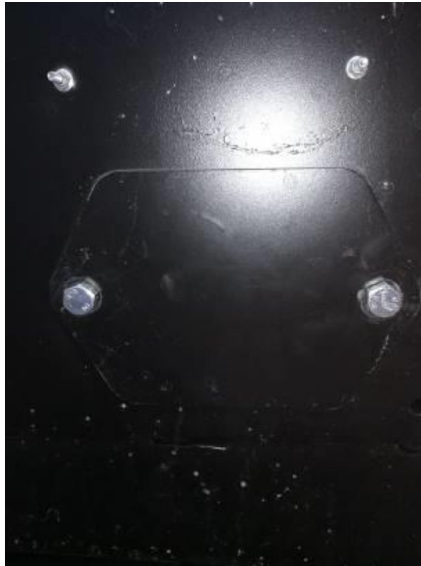
Picture 18. Hatch place
